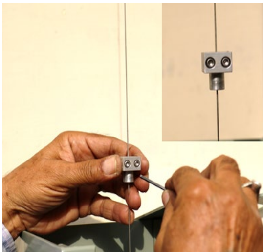
Picture 11 – fixing of top wire clamp
