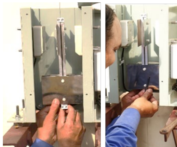
Picture 14 – fixing the plumb wire clamp at the bottom of reflector assembly
